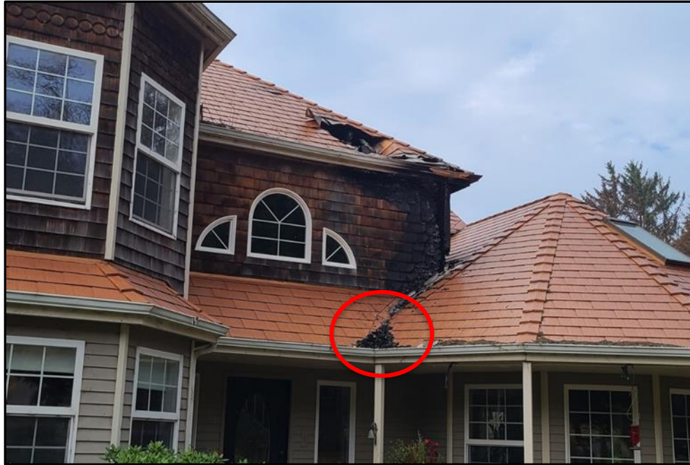
Figure 26. Attic fire started from roof/gutter debris and wildland fire (photo source: SCUF).
